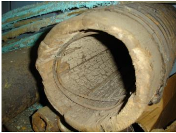
Wood Stave Pipe
