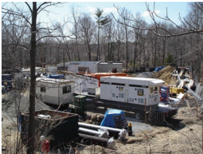
Clinton Avenue booster station construction
